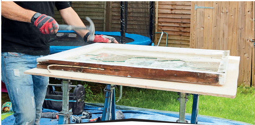
The existing float glass (which has poor heat retention) is removed.
