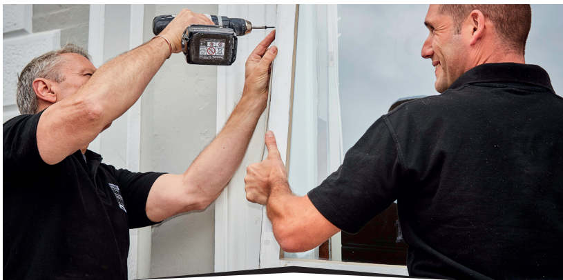
The sash is re-fitted into the existing frame.
