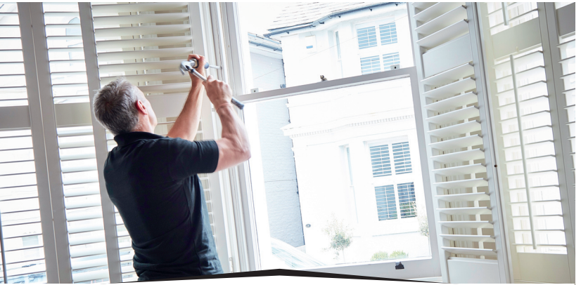
Initially the sashes are removed from the frame.
