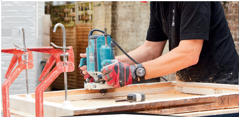
The putty rebates are cleaned and their depth is increased.
