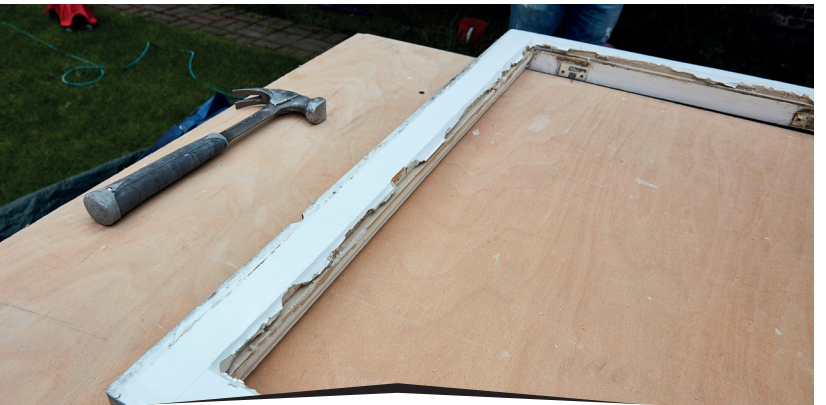
The old putty is removed.
