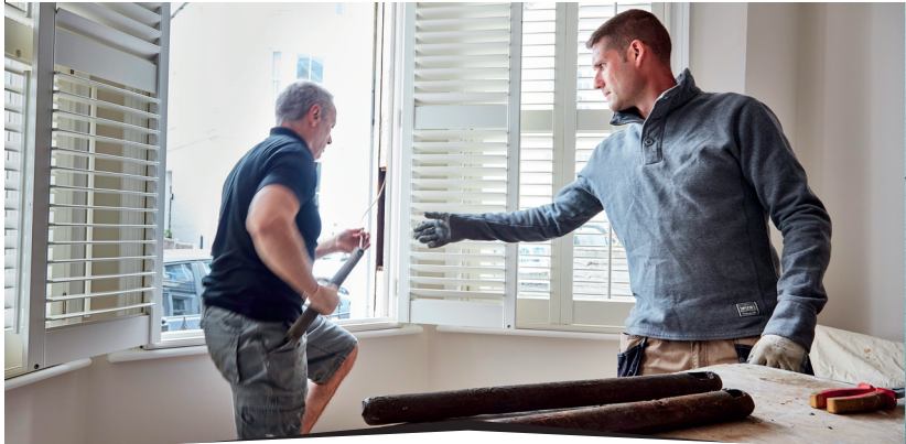
Then we remove the old cords and existing cast iron weights.
