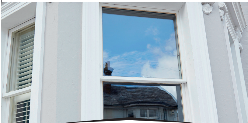
The completed project, using the existing timber windows, but with all the benefits of modern double glazing.
