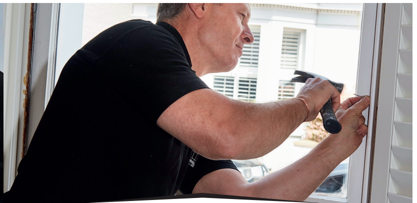
New, draught-sealed beads are installed.
